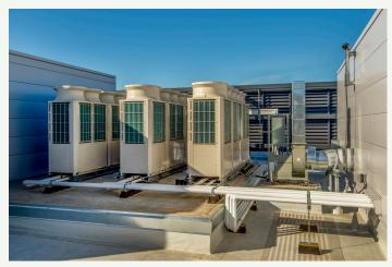
heating for another. Large distribution fans are not needed in VRF systems, nor are multiple chillers, boilers, piping, and pumps. Ductwork needs are minimal or eliminated altogether. VRF systems are extremely quiet, flexible, and provide superior load matching for increased comfort and dehumidification.
