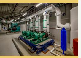
A Lawrenceville facilities manager called PJM to investigate **failed bearings** on several pumps. Frosting and fluting on the bearings indicated VFD-induced shaft voltage, so we installed shaft grounding rings on all VFD pumps and fans as an inexpensive way to protect the equipment from future bearing loss and prevent downtime.
