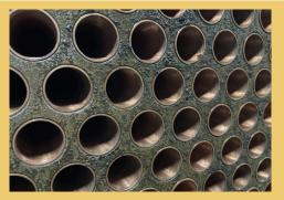
A new customer was experiencing a gradual loss of temperature in a reheat hot water system. An investigation revealed calcium buildup on the steam-to-water heat exchanger and several strainers, the result of a water softener bypass valve being left wide open. Upon removing the buildup and closing the valve, temps returned to normal.
