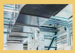
PJM was called to a large office building when a 50,000 CFM main air handling unit failed to restart after a routine filter change. A check of the control wiring traced the problem to a fire damper limit switch that was not working due to an obstruction preventing the damper from opening all the way. We removed the obstruction, checked all other dampers, and restored the system to normal operation.
